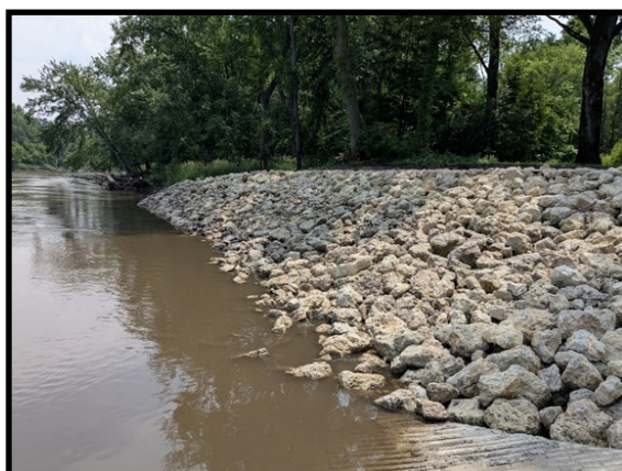
Rip rap along streambank at North Cedar Park
